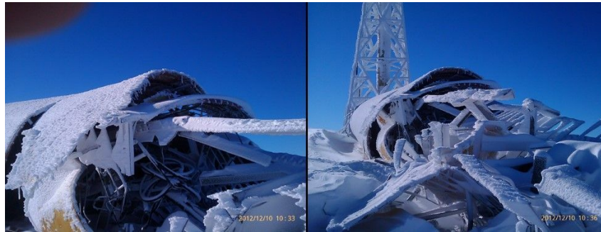
Figure 12. Remains of the collapsed tower.
